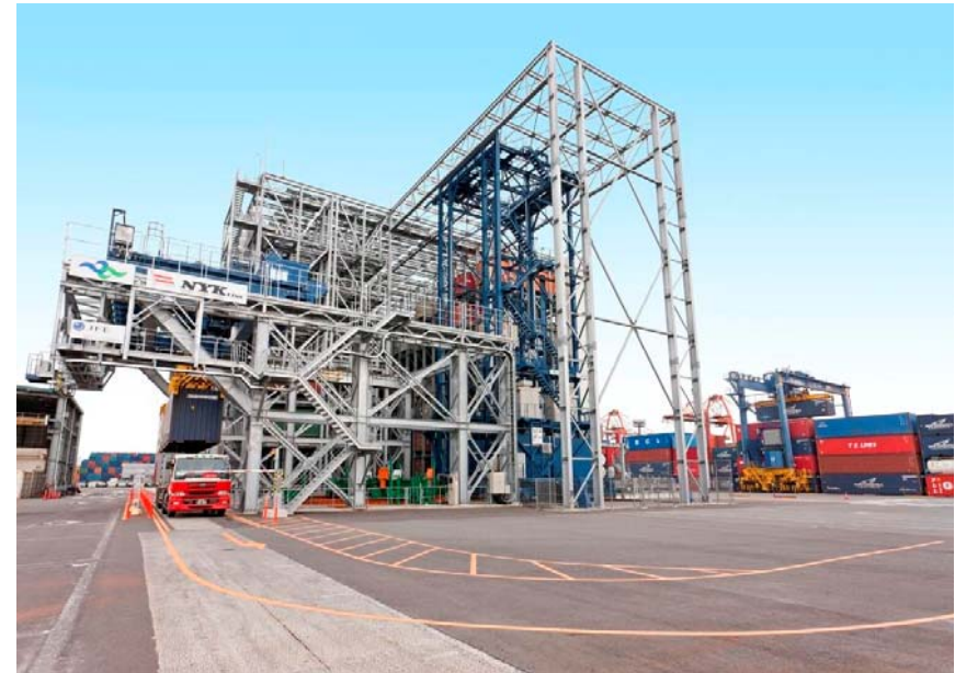
Overview of Container Hangers
